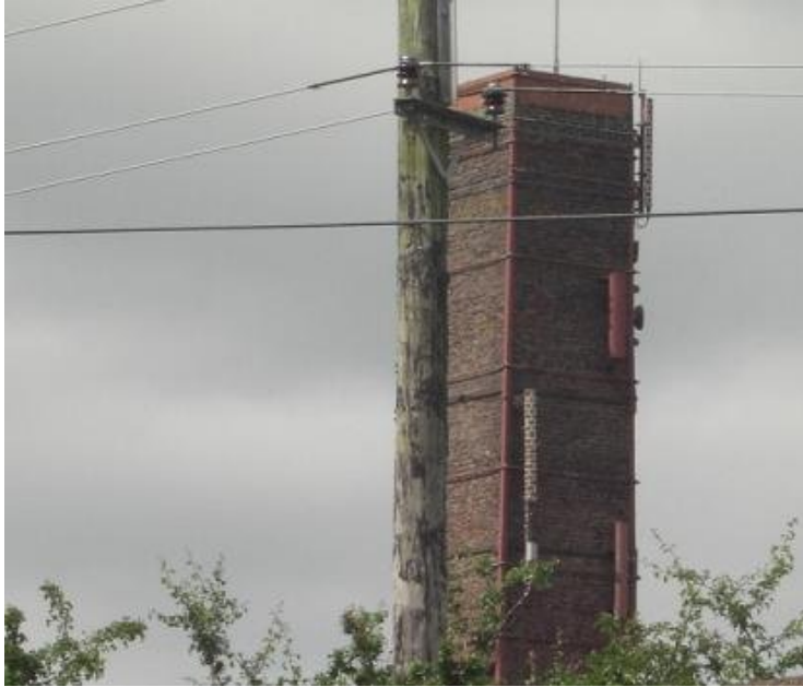
Transmitter Site Photo
